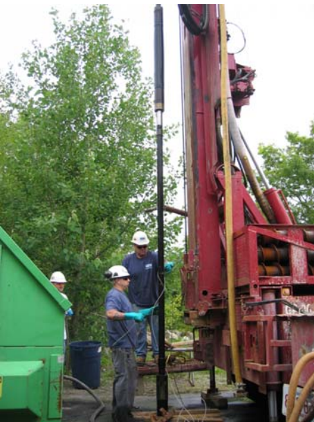
Picture 3: nZVI injection
